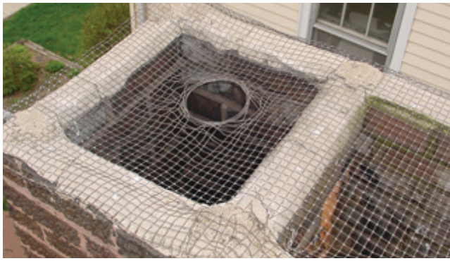
Figure 7. A raccoon made a home in this chimney after breaking through this “home-made” chimney screening. Non-professional screenings also may become packed with snow or ice thereby forcing toxic exhaust gases back into the home.
